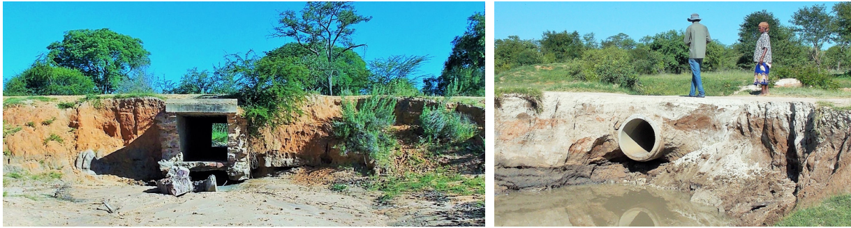
Figure 7: Two examples of inappropriately designed and seriously eroded culverts on the road near the divide, that actually overtopped during a flash flood early in the 2020 rainy season. All smaller fish and most larger fish would have great difficulty getting across these obstacles
